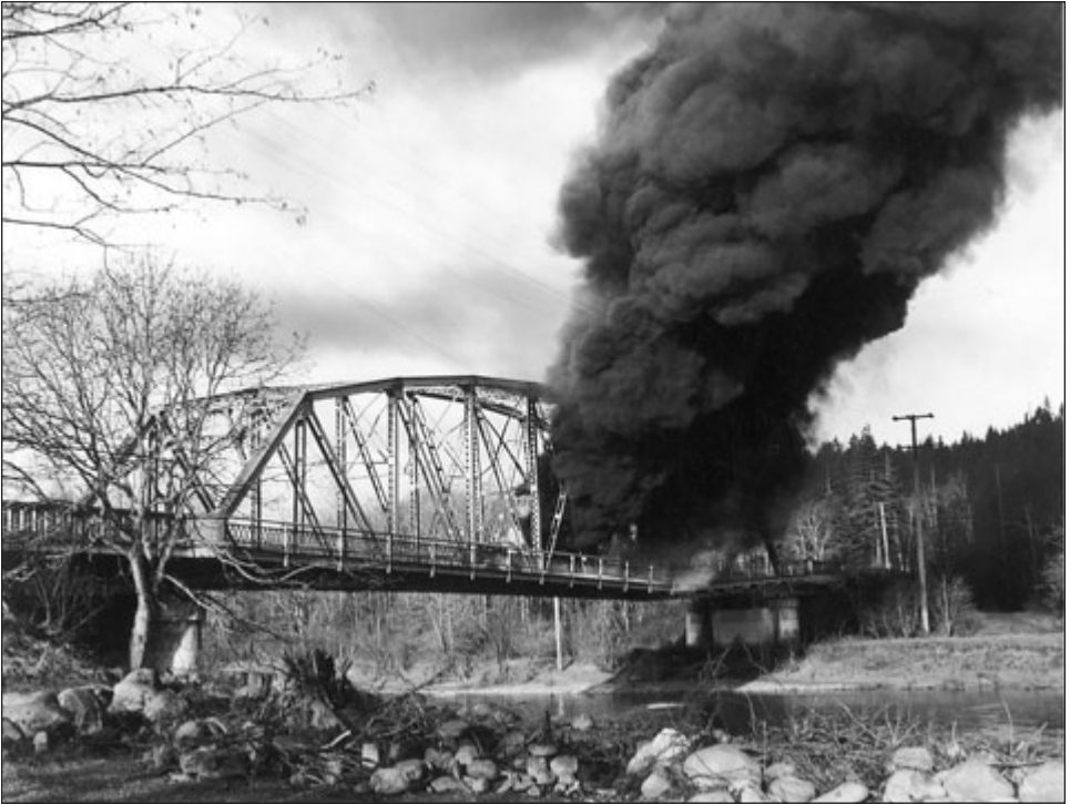
Bridge in the vicinity of Marignane.
